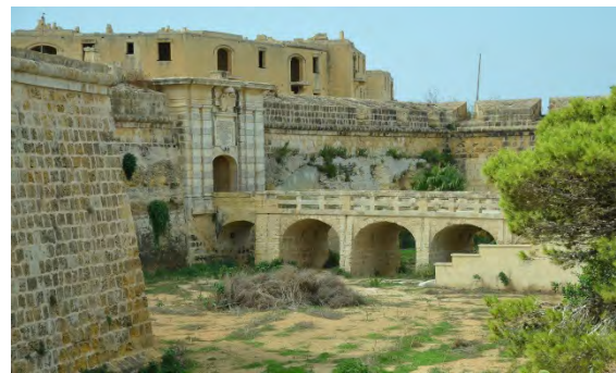
Fig. 24: The main entrance to the Chambray fort, which is now impassable, with an investment ruin in the background.
