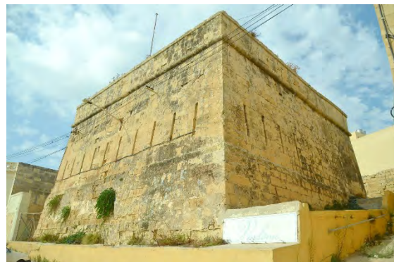
Fig. 33: Bulky emerging outer walls with narrow niches of the Vendôme-Redoubt.
