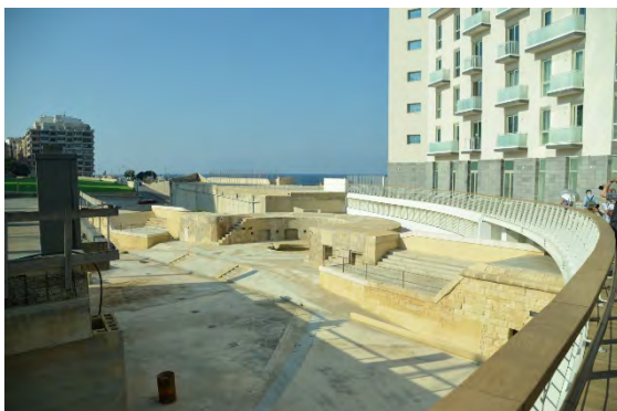
Fig. 12: The garden battery is pushed out of the underground high-rise complex.
