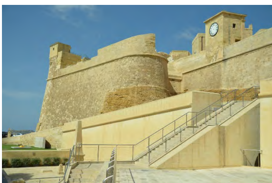
Fig. 26: Under the stairs in front of the half-bastion St. Martin of the citadel in Victoria is the entrance to the visitor center.
