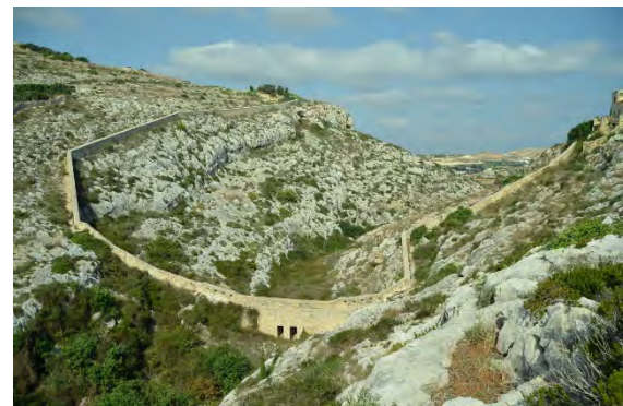
Fig. 27: The barrier wall at the beginning of the Victoria line with culverts in the valley floor.
