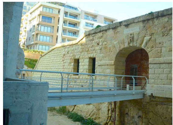
Fig. 14: A modern department store center is hidden behind the historic facades of British barracks.
