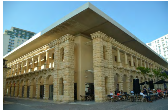
Fig. 13: The best view of the entrance gate of the Cambridge battery could only be seen from the underground car park
