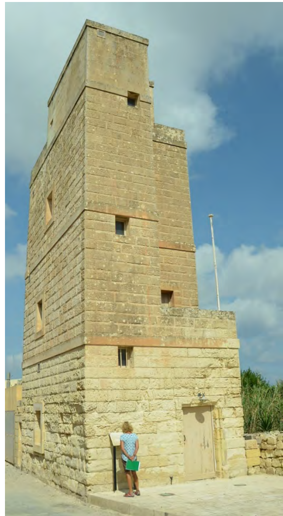
Fig. 29: The refurbished semaphore tower in Gharghur, which was once built for the purpose of telegraphic transmission.
