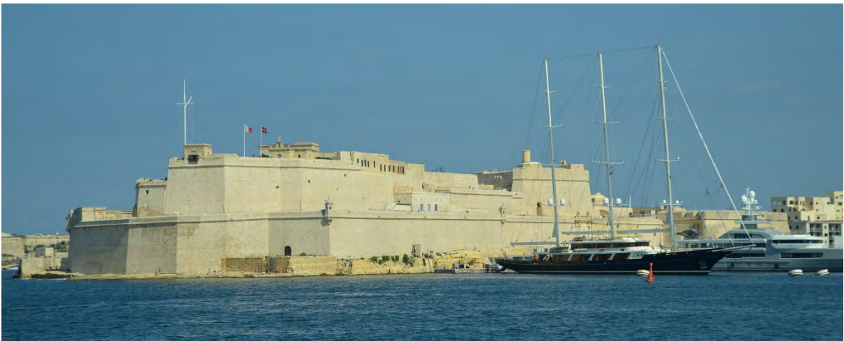
Fig. 06: View from the ship to the sea-side access side of the Angelo fort.
